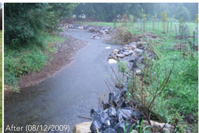
Figure 8.1.2 Example of stream bank stabilization, showing how extreme measures (e.g. use of rock) is sometimes needed to stem erosion and loss of sediment in cases where upstream sources of stormwater runoff are not also curtailed. Photo credit: USDA-NRCS-New Jersey.
