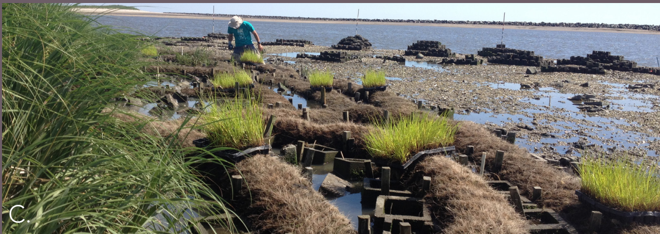
Figure 5.2.9 Hybrid living shoreline concepts of DELSI: A) utilizing oyster shell bags to attenuate problematic boat wakes at Matts Landing, Maurice River, NJ; B) A mosaic of shell bags and oyster castles were installed to attenuate waves and provide substrate for oysters to improve water quality, at Nantuxent Creek, NJ; and C) Planting smooth cordgrass on coconut fiber logs (foreground), which were coupled with oyster castle pods (background) to expand the existing oyster reef footprint to improve water quality as well as attenuate waves at the Mispillion River Inlet, DE.
