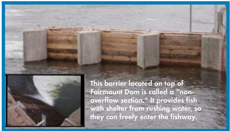
Credit: Philadelphia Water Department
