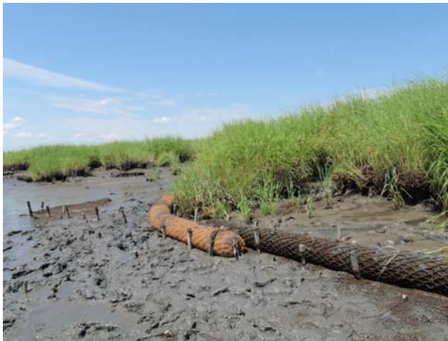
Installations of “living shorelines” like these on the Maurice River, NJ can help prevent erosion of wetlands.
